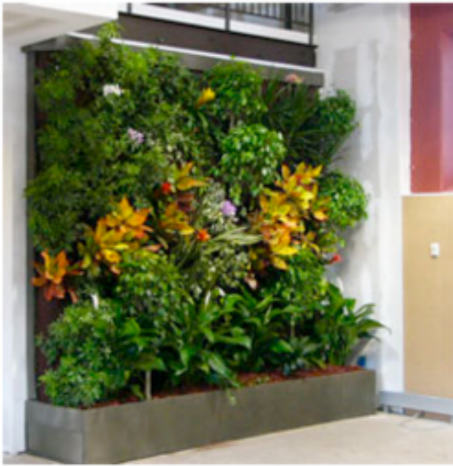
Living Wall installation, Baltimore, MD. This 110 sq ft (10 sq m) wall filters all the air for its 7,500 sf office building. Notice the ornamental character of some plants chosen
