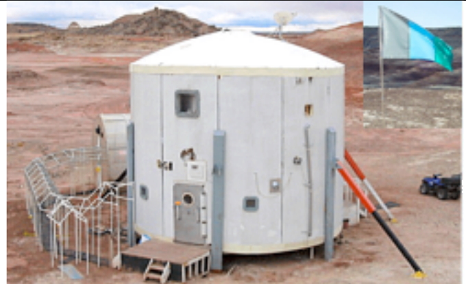
Mars Desert Research Station, Hanksville, Utah, site of the Moon Society Simulation Exercise on Crew 45, Feb. 26 – March 11, 2005, showing the simulated tunnel structure that we built between the Hab and the GreenHab.
